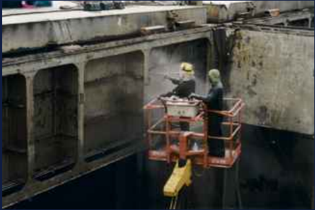
Decontamination of the Choyang Success after fire damage.
